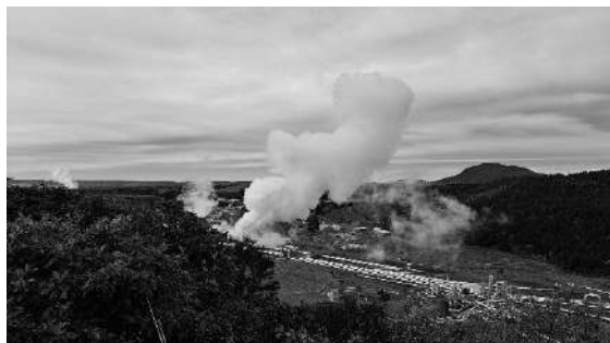
■Wairakei Power Station
