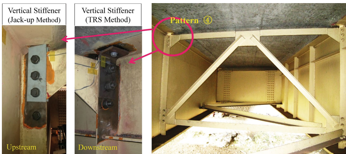
Fig. 6. Sway bracing connection retrofit
